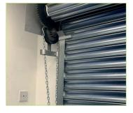
The shutter is operated via a haul chain system, assisted by a springloaded barrel, providing a counterbalance to the weight of its curtain, making operation easier
